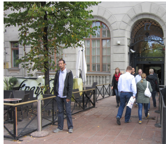
The area has been defined using open fences (under 90 cm in height), made with steel structures. Access to the building has been taken into account.
