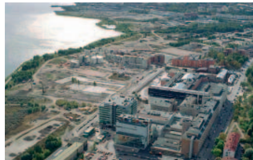
Figure 5. Area in 2004 under construction.
