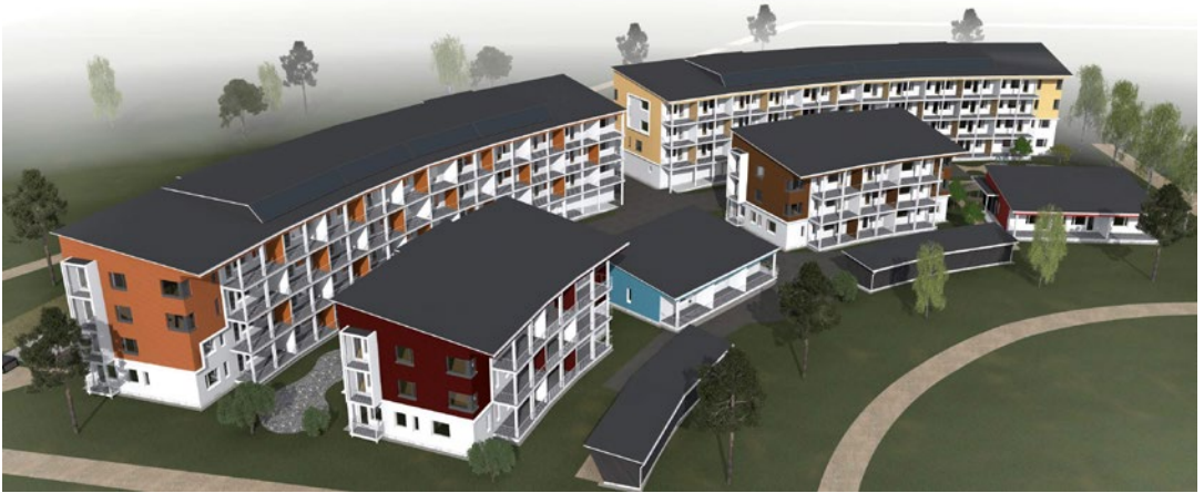
In Honkasuo residential district, wooden construction has been combined with high energy-efficiency.
