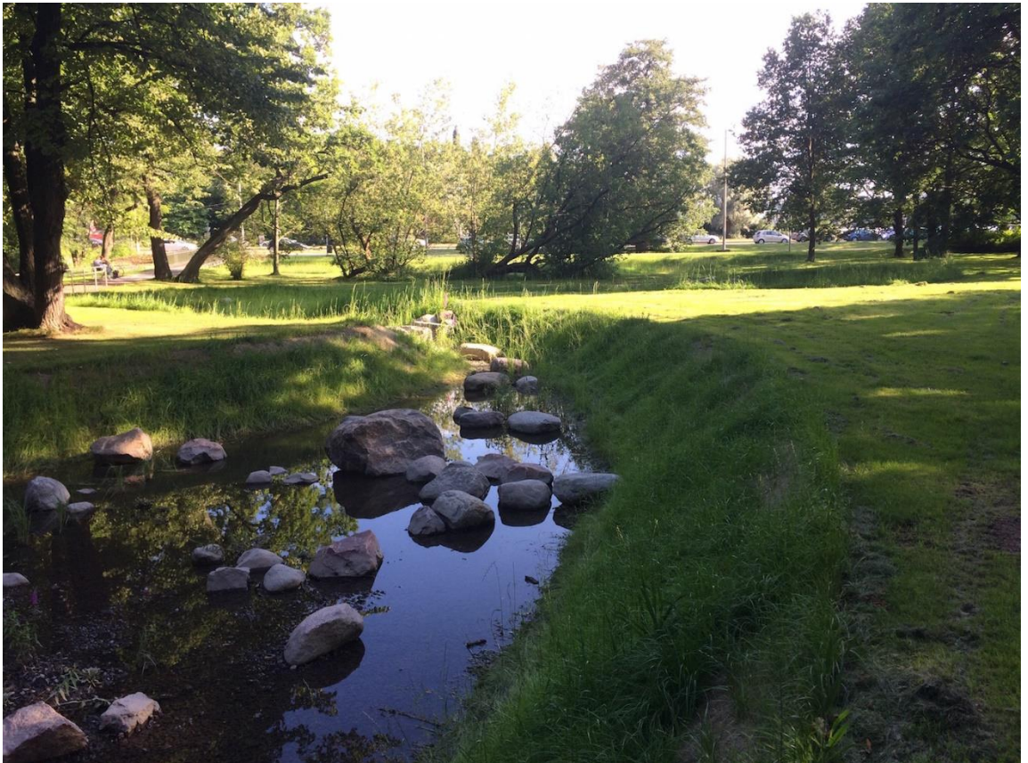
Image 3. Töölönlahti wetlands, which will retain and clean stormwaters flowing from the direction of Pasila. Photograph by Elisa Lähde.
