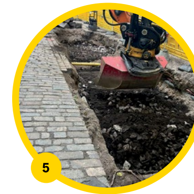
Structural soil renovations (17m 3 )
