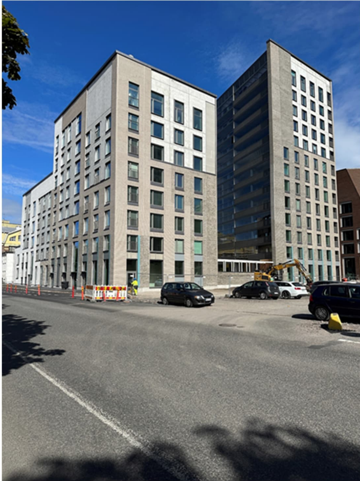
Figure 12: EXCESS demo building in Kalasatama, Helsinki, December 2024.
