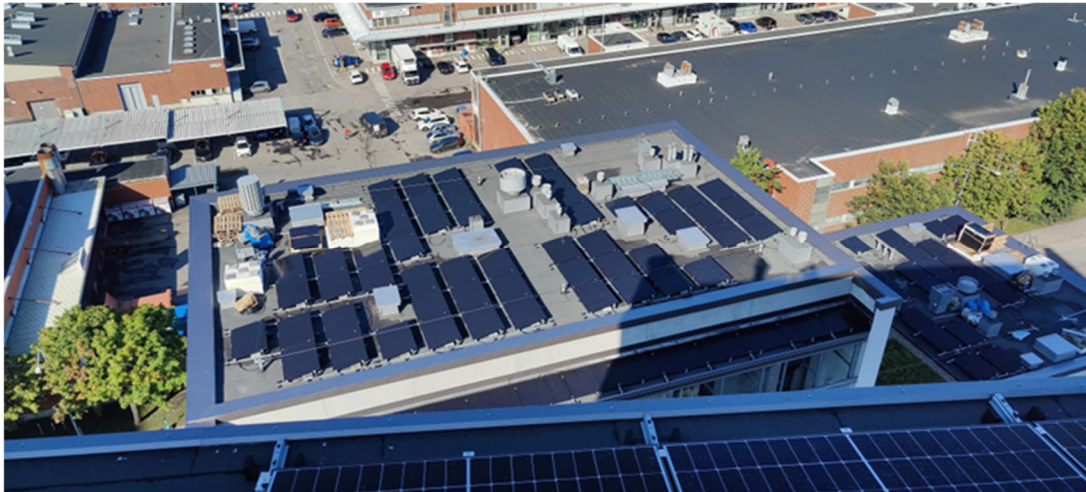
b. PVTs at roof, general view
