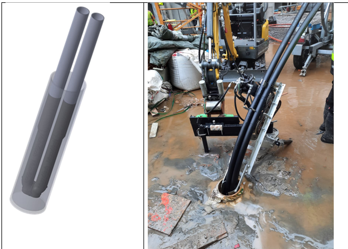
Figure 16: BHE TC55 designed for semi-deep boreholes(SDR17/SDR11)
