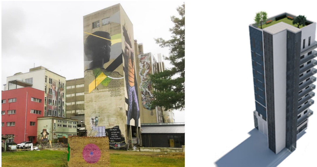
Figure 4: Original state of the feed production silo tower (left) and 3D rendering of the planned refurbishment (right)
