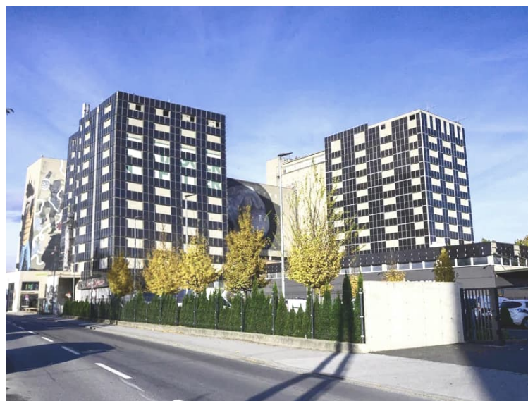
Figure 3: View on the partly transformed industrial area from the south, showing the EXCESS demonstration building no. 10 to the far left
