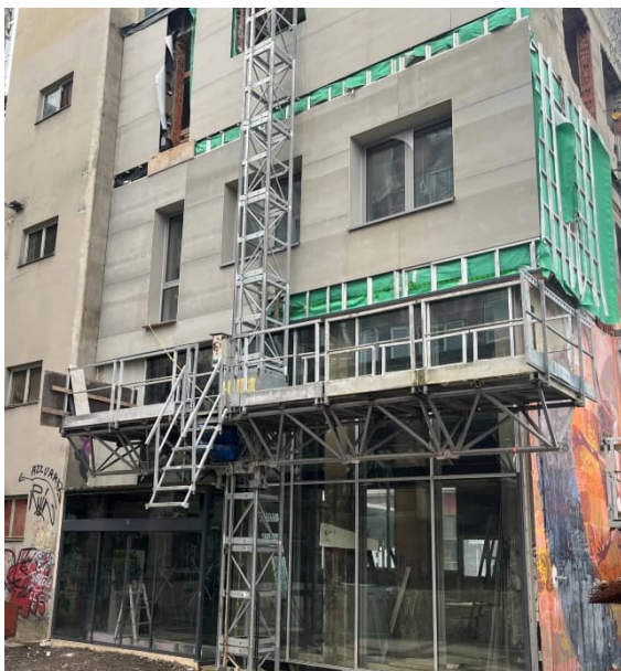
Figure 8: Partly installed multifunctional facade modules at the Austrian demonstration building
